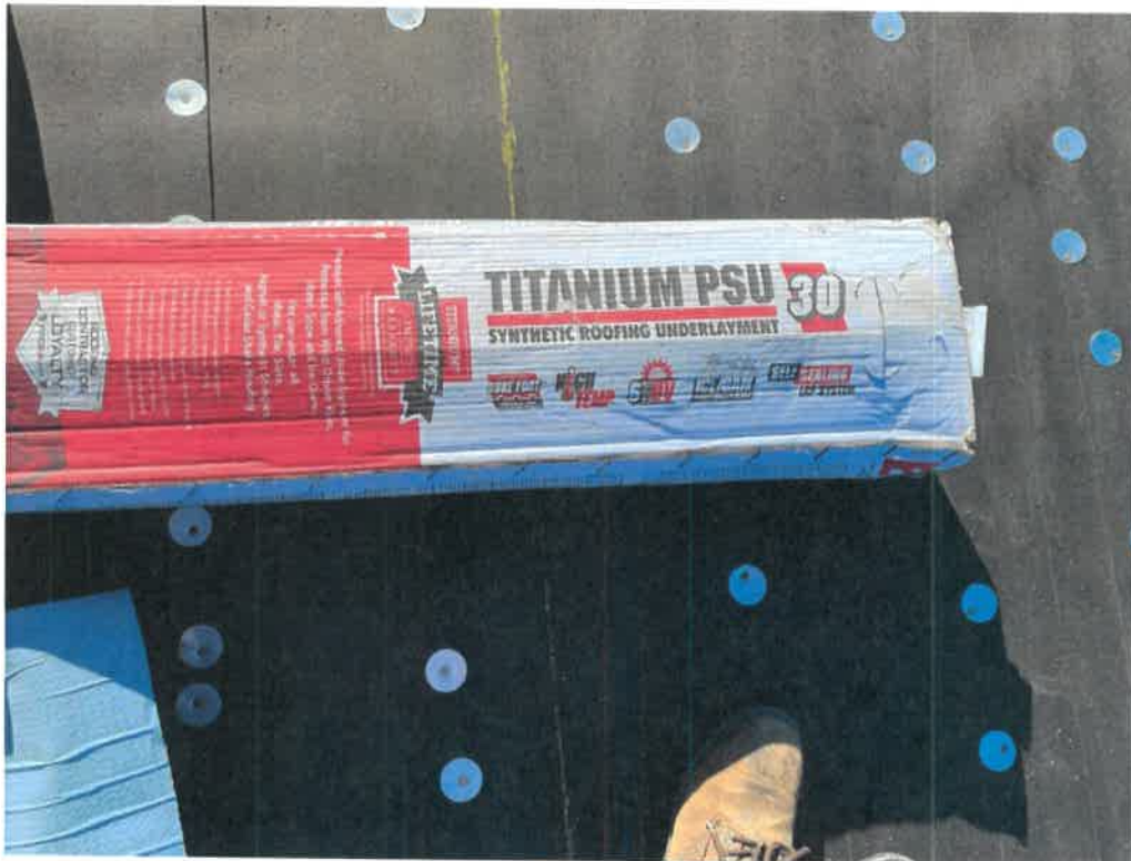
Figure 4 – Secondary Water Barrier at Sloped Section (Typical)
