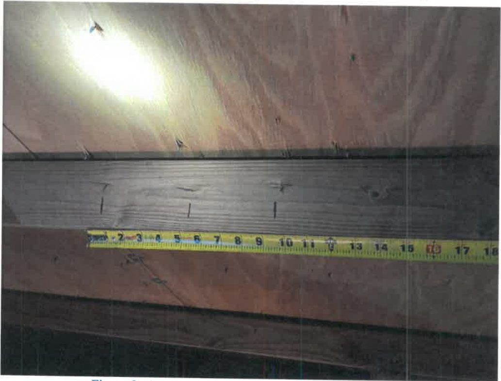
Figure 2 – Plywood Sheathing Fastener Spacing (Typical)
