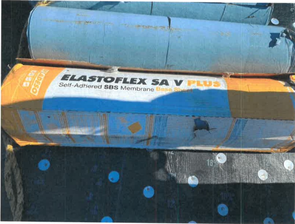
Figure 5 - Secondary Water Barrier at Flat Section (Typical)
