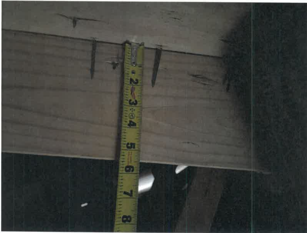
Figure 3 – Sheathing Fastener Size 8d Confirmed (Typical)
